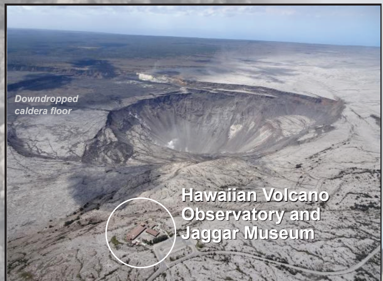
The USGS Hawaiian Volcano Observatory and NPS Jaggar Museum on Kilauea's caldera rim were vacated in mid-May 2018 due to earthquake damage associated with summit collapse events. As of June 2019, HVO staff are in temporary office space in Hilo. Jaggar Museum remains closed.
